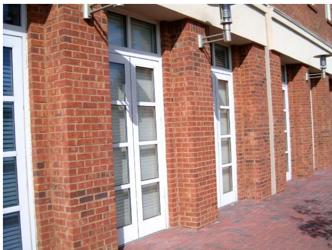
Street level windows closed with no displays
