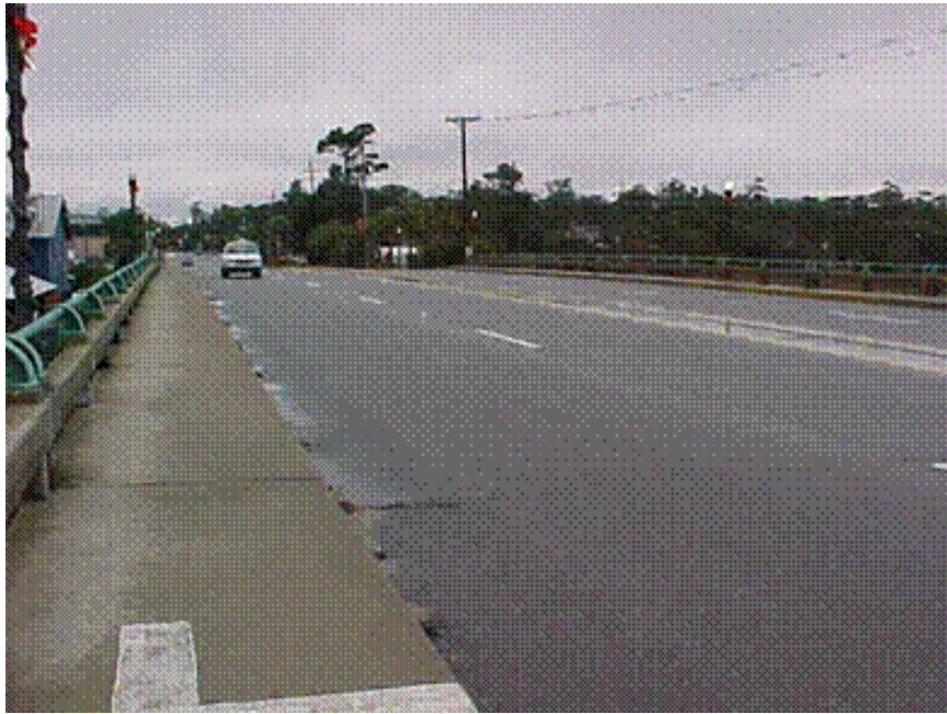
Shem Creek Bridge
